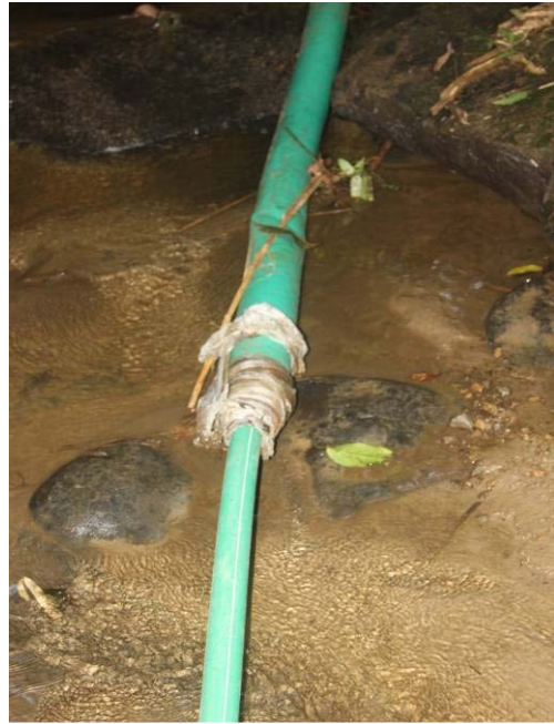
Picture 35: Joint fitting with workable materials
