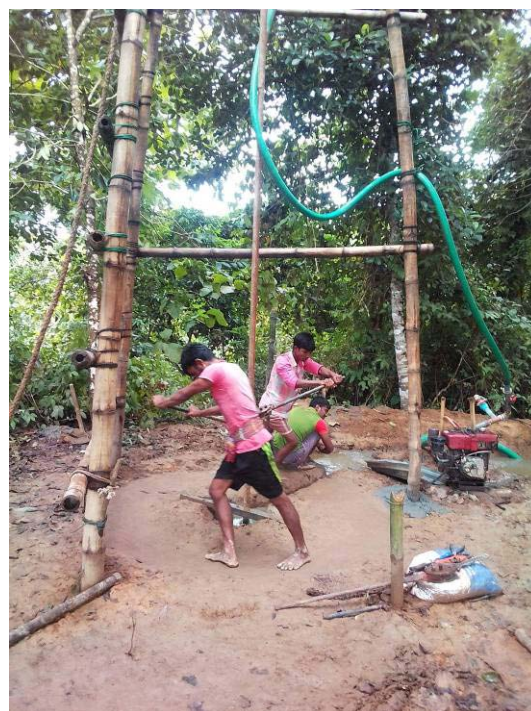
Picture 45: Deep set tube well installation on the ground of Sogodasori Community School by the hired team of plumber
