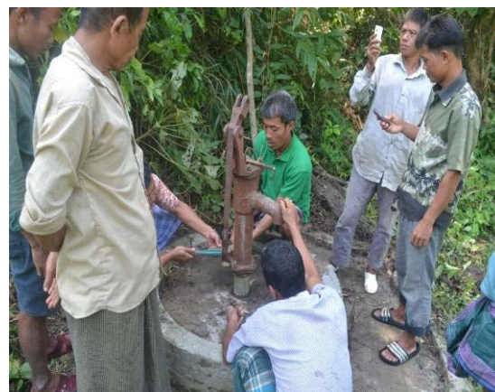
Picture 47: Local technician repairing the ring well in assistance of the communities
