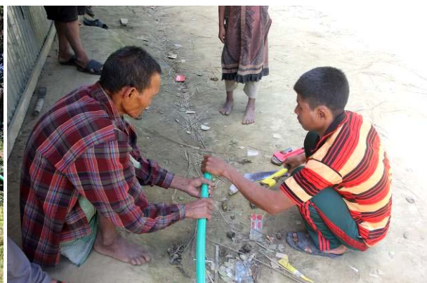
Picture 38: Trained local armature technical resource trying to join pipe lines
