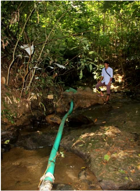
Picture 34: Water collection point of Perasora School GFS located more than four km. Away from the reservoir
